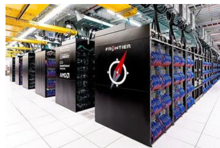
Credit: Data Centre Dynamics
